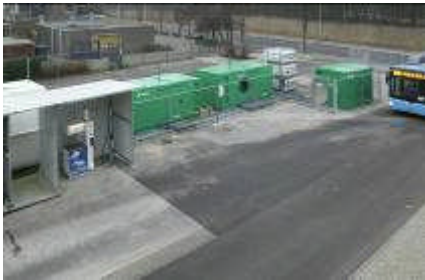
Ede, Holland Bus depot Gas Station
