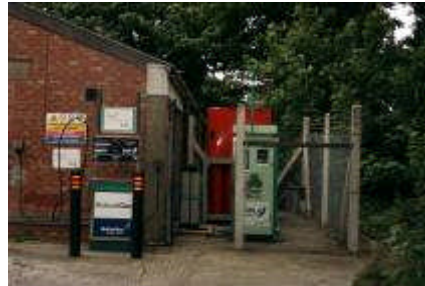
Bournemouth Council Gas Station
