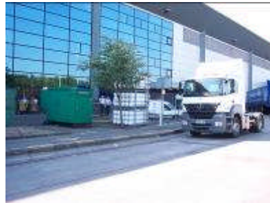
Tesco Middlewich Trial Gas Station
