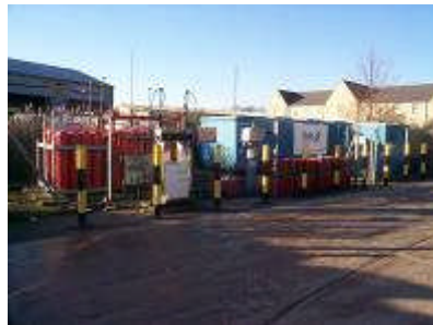
W.Oxfordshire Council Gas Station
