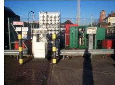
Northampton Bus depot Gas Station
